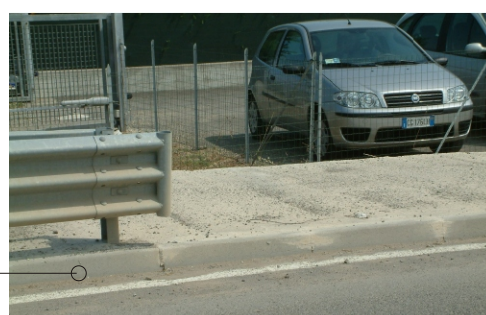
Cordolo, marciapiede in cemento e guard rail
